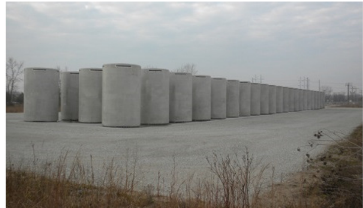
NAC MAGNASTOR spent fuel casks on the Zion ISFSI pad.
